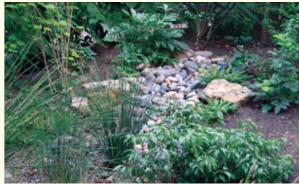
There are a number of ways to move the water from the downspout to your rain garden. This homeowner uses a dry streambed that is lined with plastic for the first few feet near the foundation. The downspout pipe is hidden by rocks and plants giving a more natural appearance. The rocks also slow the stream of water to prevent erosion.
